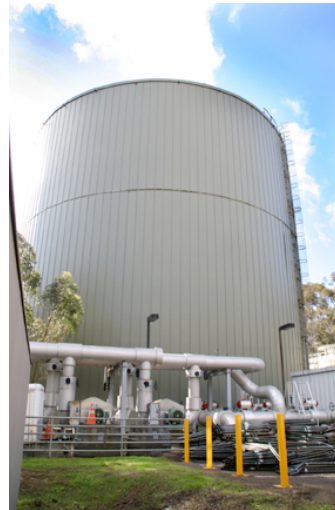
Cold Water Storage Tank
