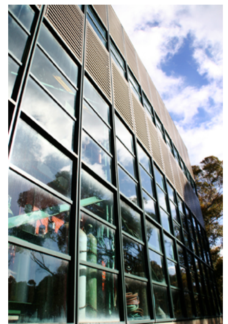
UC San Diego Central CHP Plant
