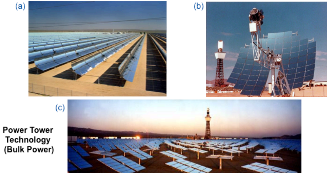
Figure 12.2: Photographs of (a) linear parabolic trough array, (b) parabolic dish and (c) power tower SEG power plant configurations.
